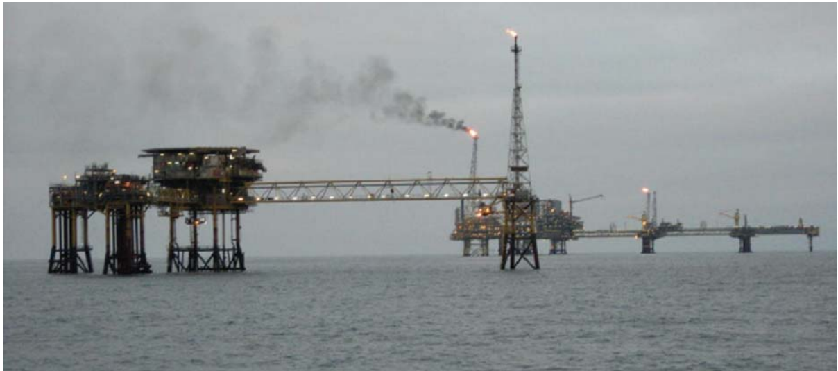
Fig.1 The Dan Bravo Oil & Gas Platform in Northern Sea (Mærsk Oil & Gas A/S)
