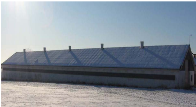
Fig.1 Testing Facility in Syvsten, Denmark
