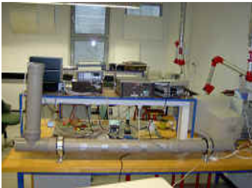
Fig. 1. ANC benchmark – Ventilation Duct in AUE
